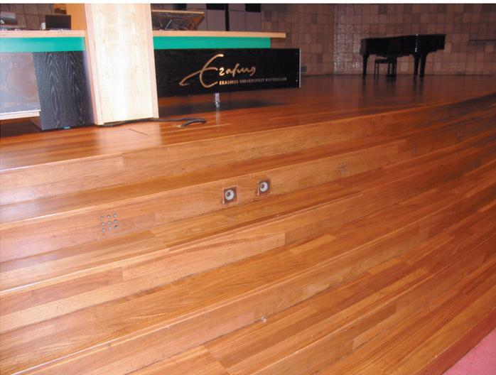
*The front fills, nine speakers total, were mounted into the staircase structure. The protection grids are very solid because shoe tips are close and legion. The vents left and right to the miniature loudspeakers don't have anything to do with the sound system.*
